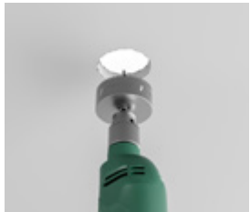
Make a hole with a standard 80 mm hole saw
